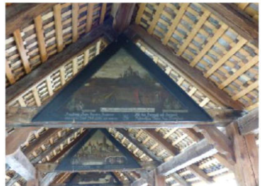
Painting in the bridge eaves.
